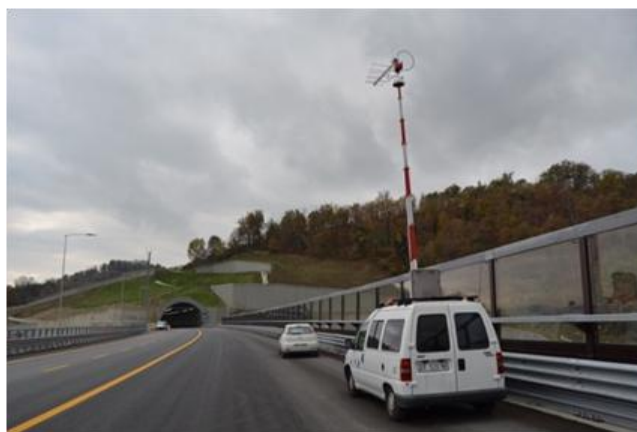
Figure 2: Puliana tunnel, example of external transmission
