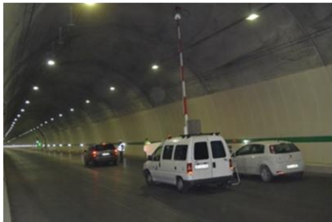
Figure 1: tests in "Base" tunnel without traffic
