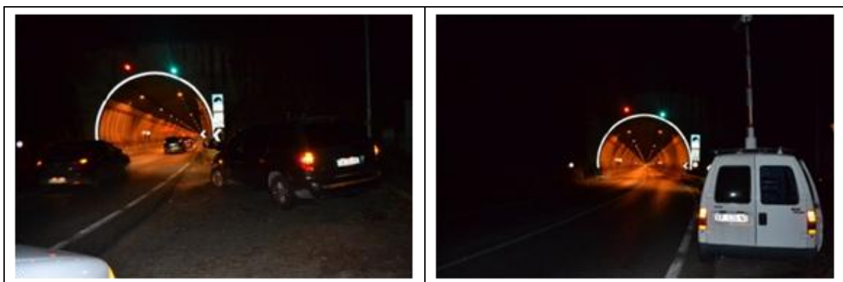
Figure 7: “traforo del Pino” tunnel (SP10) with and without traffic
